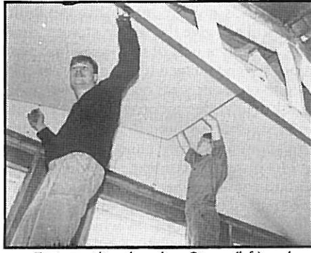
Fitting ceiling boards - Simon (left) and Stephen from the MSC team.
