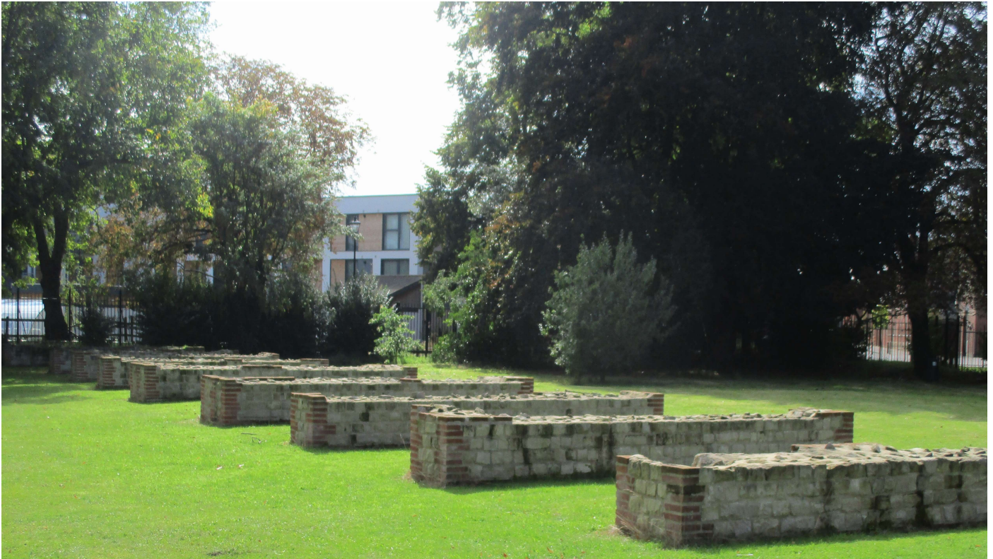
600mm-high wall stumps built immediately above the actual Roman foundations of the starting-gates, made from stone and 'Roman' bricks. Photo: Michèle Abson
