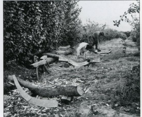
Above Left: Halving an oak log vertically, Saxon style (West Stow 1998)
